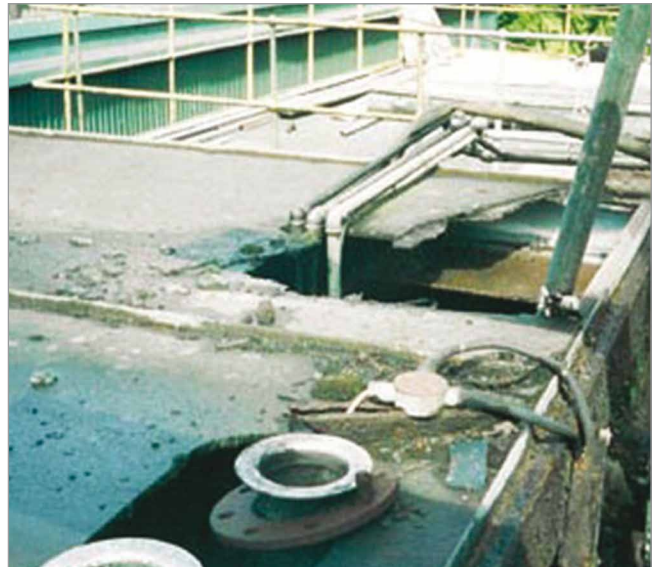
Tank roof corrosion
