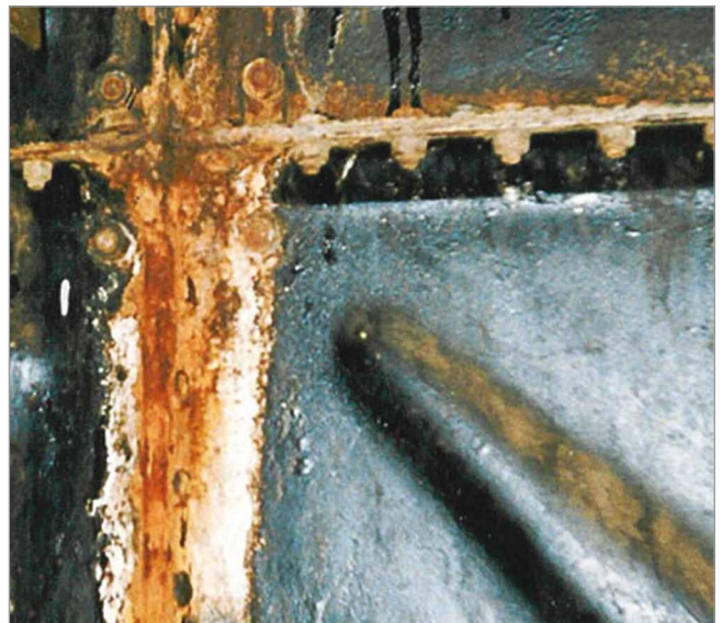
Failed joints causing leaks and corrosion
