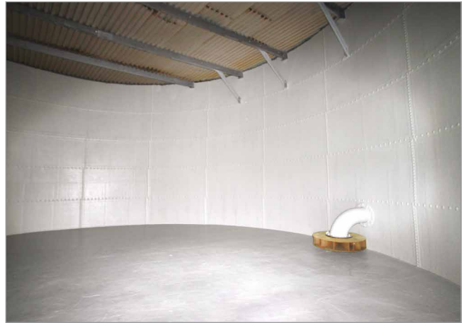
For a firewater sprinkler tank - refurbishment to inside walls and roof purlins.
