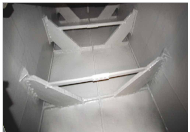
Potable water storage tank.
