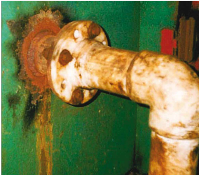
Pipe connection corroded and leaking
