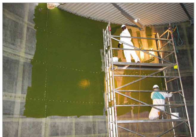
Completing a tank GRP lining.
