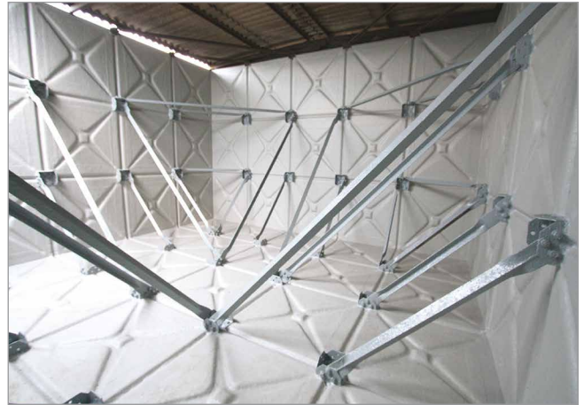
Sectional Braithwaite water storage tank.
