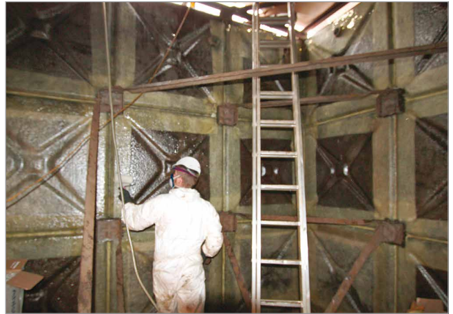
Application of GRP lining to a sectional water tank.
