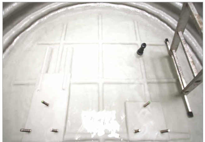
Repairs to an underground effluent tank, damaged due to pressure from the water table.
