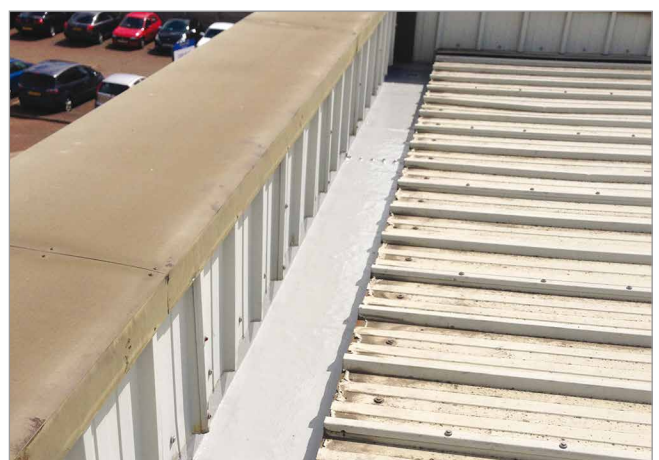
Roof Gully Lining
