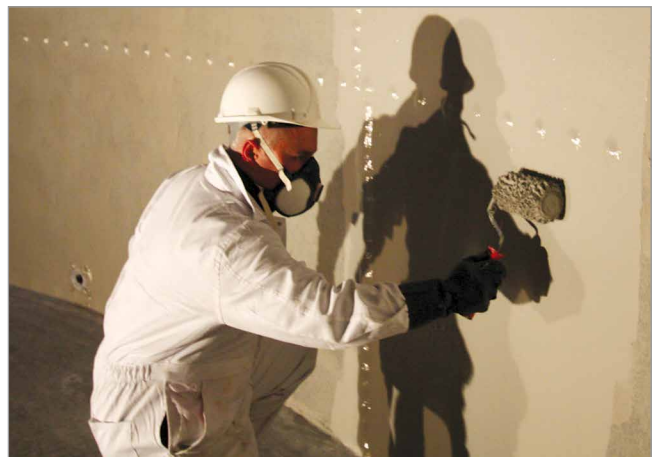
Completing the top coat for a tank GRP lining.
