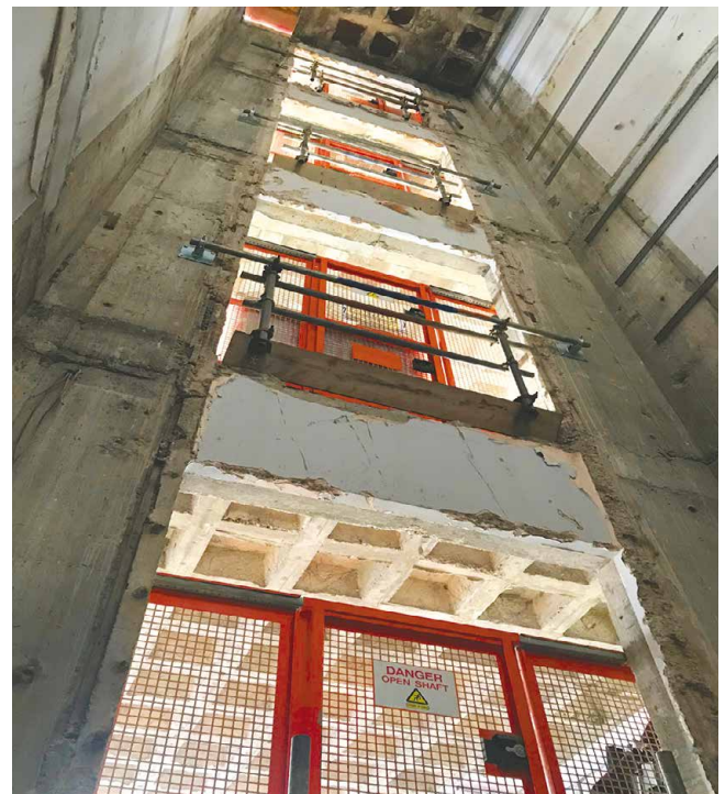
Riser shafts prior to GRP mesh flooring.
