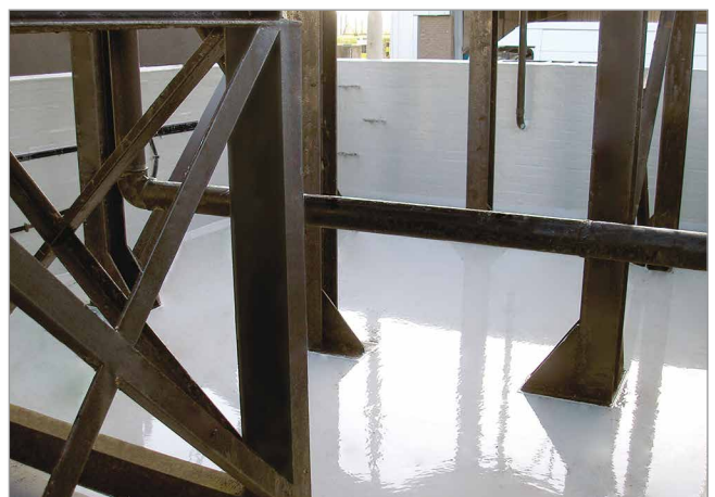
Oil bund. The GlyCol bund life was extended with addition of a GRP lining.
