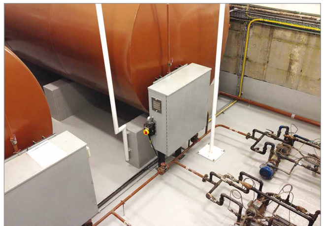
Generator bund. GRP lining, including internal concrete trench runs, complicated pipe and cable areas.
