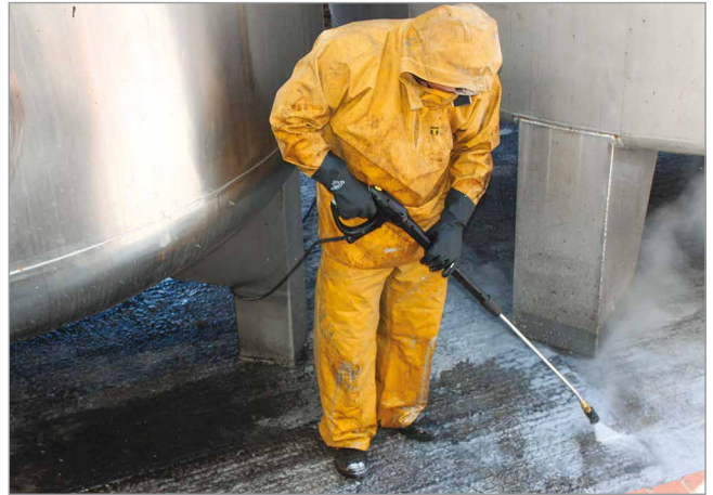
Bund lining preparation. Pressure washing prior to cleaning, gritblasting and application of GRP lining.
