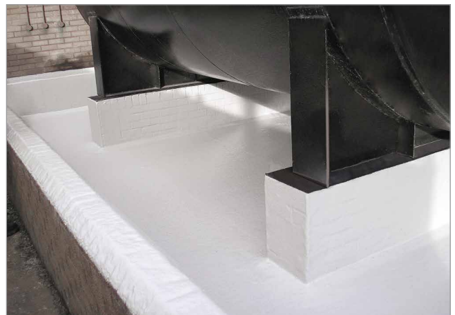
Aviation fuel tank bund areas with completed GRP lining.
