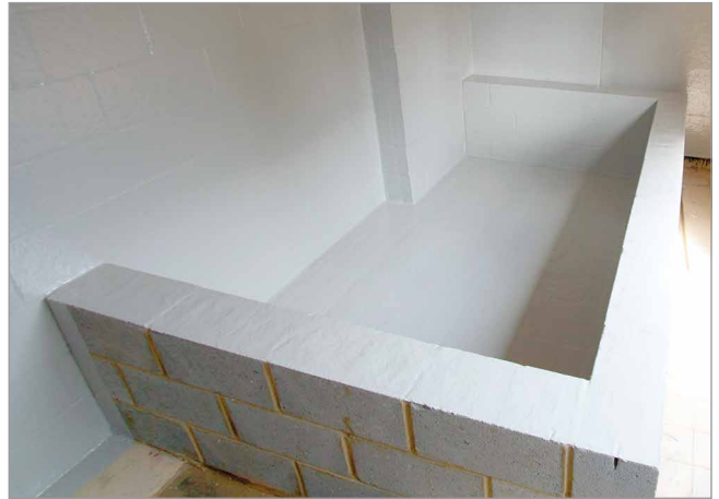
Water and waste water. GRP lining for a water and waste water management company acid dosing room.
