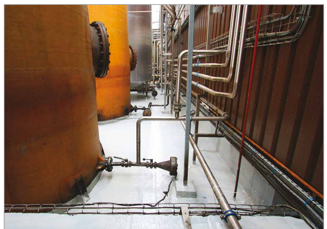
Tank bund. GRP lining of storage tank bunds and pipe areas for a food preparation factory.
