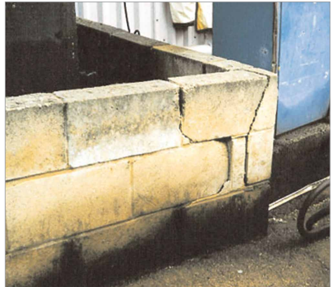
Damaged bund wall
