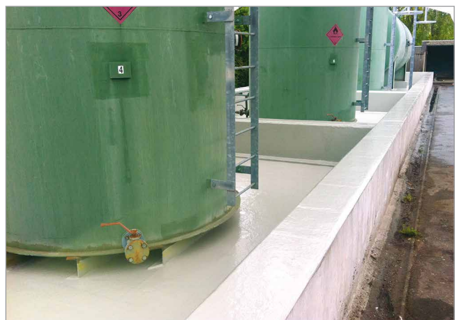
3. Completed, a GRP lining creates a new bund within the existing structure.
