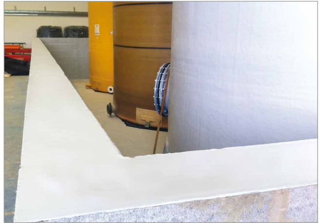
Chemical storage bund. A GRP lining installed to a new internal silos bundled area to maximise the bund life.
