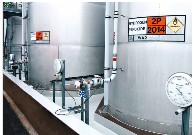
Hydrogen peroxide storage tank bund.
