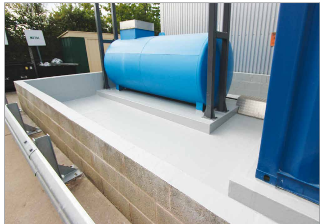
A tank bund impermeable bund lining added within a week.
