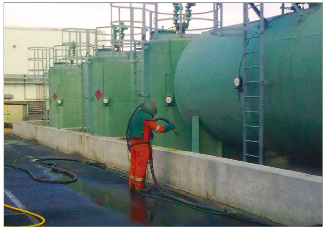
1. Surface preparation to remove foreign matter.
