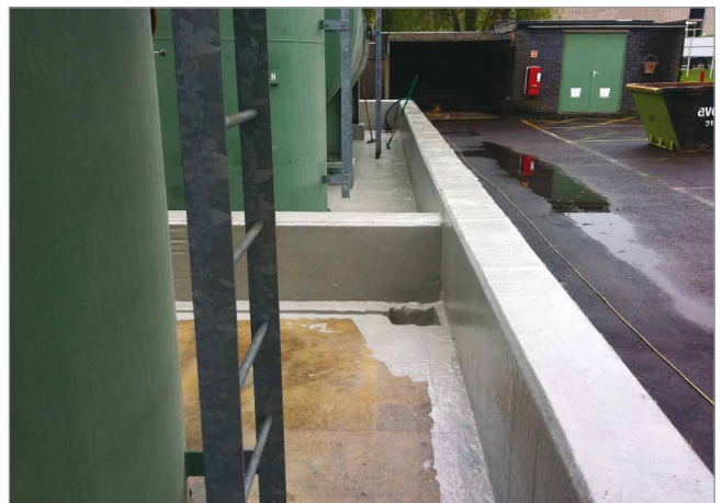
2. A 4-coat lining system is applied to the existing structure.
