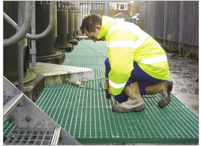
Industrial GRP grating installation.
