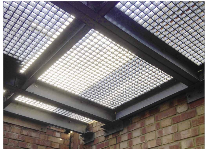
GRP grating mezzanine floor construction.
